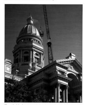
The peak of the dome is 146° high and 50° in diameter. It is gilded with 24 carat gold leaf and has been gilded five times. The first time (in 1900) three layers of gold leaf were added one over the other on the original 1887 copper. In 1979 the original copper sheeting was removed, gold leafed in a shop, and then installed on the dome. The dome was leafed again in 1986, as is shown above.
